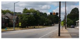
Pedestrian Hybrid Beacons stop automobile traffic for bicyclists and pedestrians wishing to cross a high traffic volume/high speed roadway.
